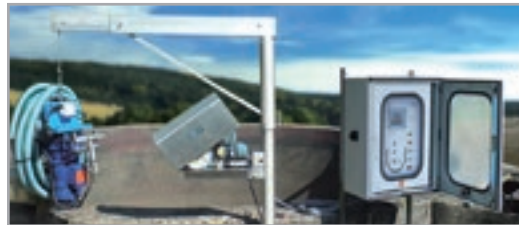
Suction entity, swiveling boom with covered gear box and control unit with touchscreen
